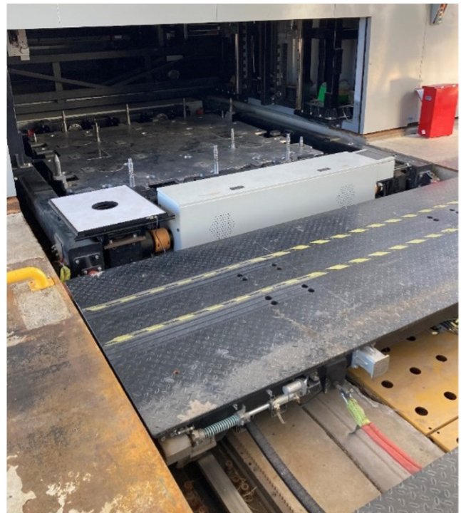
Swapping station DeepWay trucks, swapping from below
