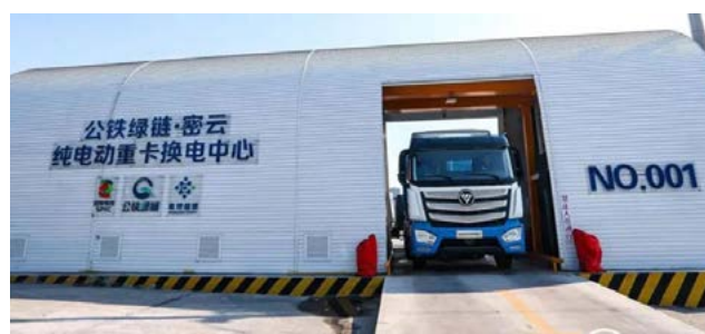
Figure 28: EHT battery-swapping station at Miyun, Beijing.
